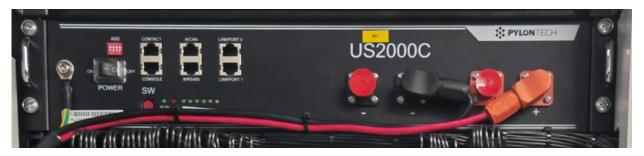
Turn on the Power switch of US2000C. Press the "SW" button of US2000C for about 3 seconds, and observe the indicator light of the UPS host. If there is mains power, the indicator light is green, indicating normal startup.
